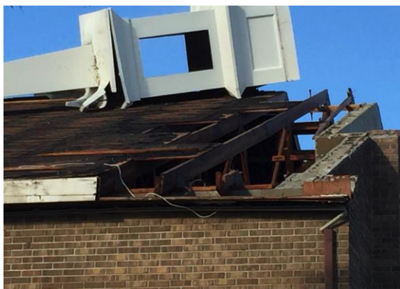
Base of the Roof system
