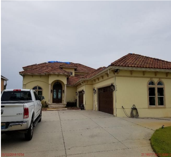
4.1.2 Street side overview
