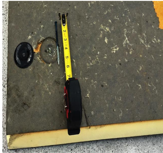
Fastener and insulation
