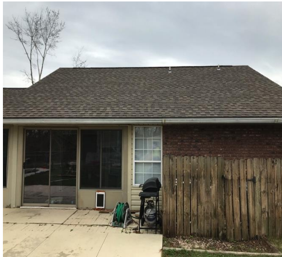
Rear of residence
