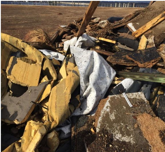
4.2.5 Fastener: it appears it was never attached to the roof deck or a nailer.
