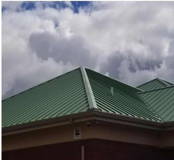
3.2.4 No roof damage
