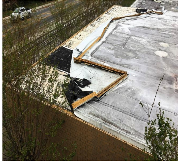
Membrane attached to nailer that was nailed to a vertical board
