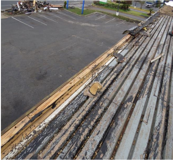
1.1.3 Original perlite was strip mopped to the deck with irregular pattern
