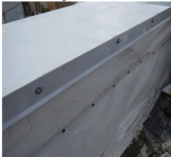
Coping and termination bar
