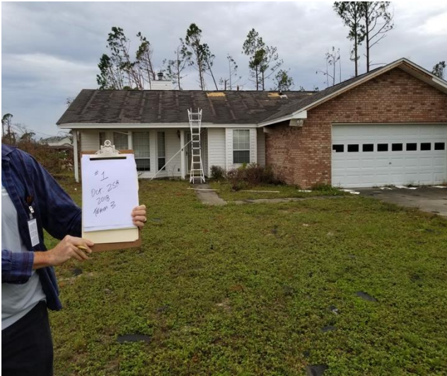
3.1.1 Overview of front showing racked shingles
