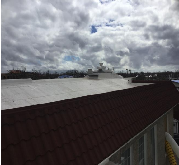
4.2.4 Overview of Barrel Roof
