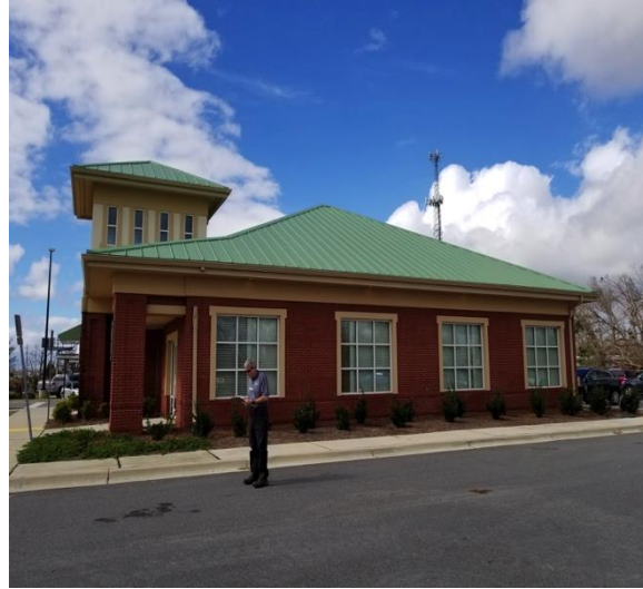
No roof damage
