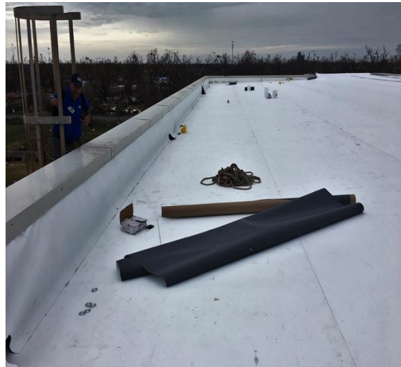
Temporary cover of upper roof
