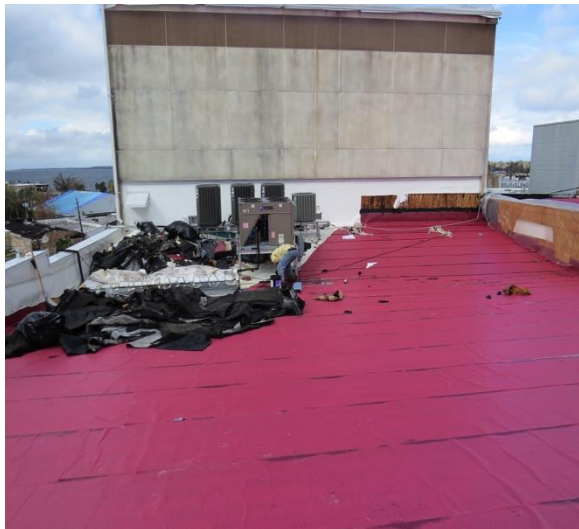
1.2.2 Overview Red temporary roof
