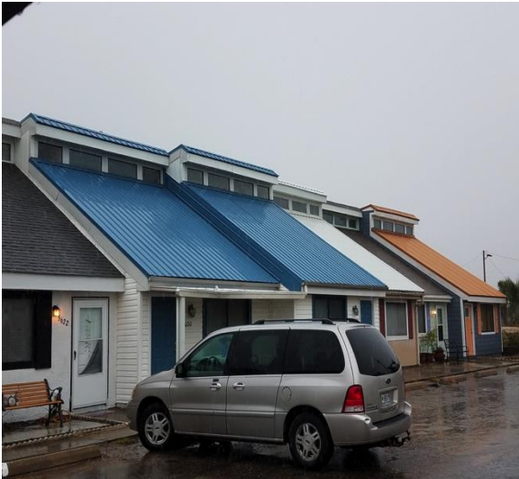
4.1.5 Interesting set of several roof types
