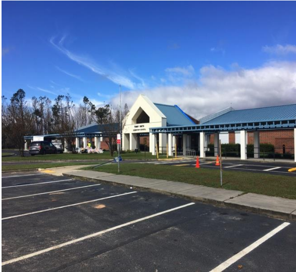
2.2.2 Overview of large complex with Standing seam metal panels
