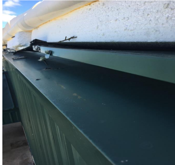
Metal edge detail that was opened
