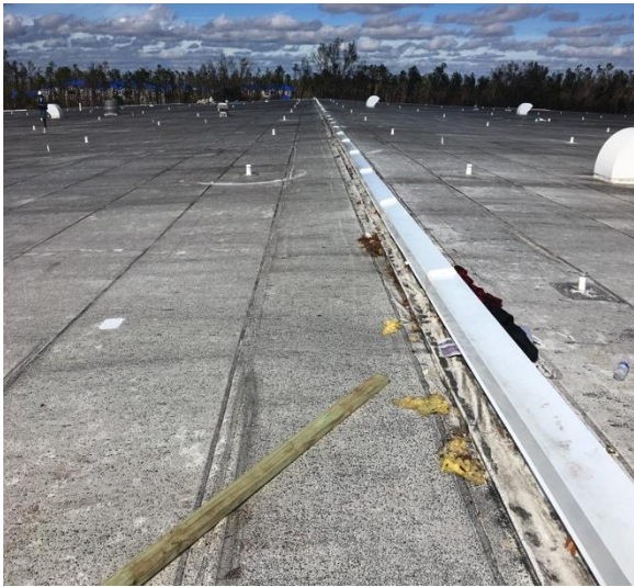
2.2.4 Overview of large roof
