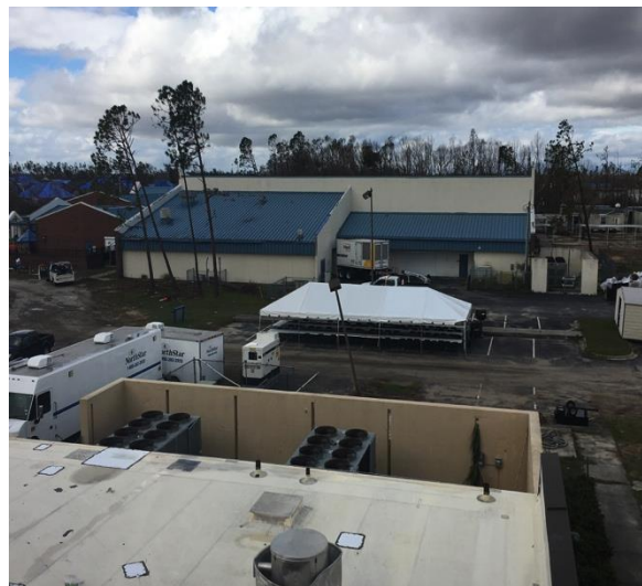
No observed damage on other sections
