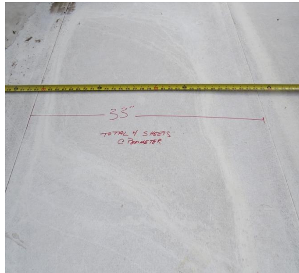
Half sheets at the perimeter
