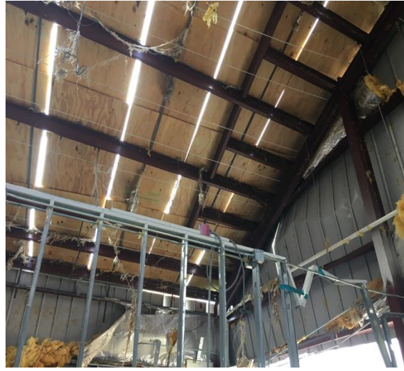
Wall side interior
