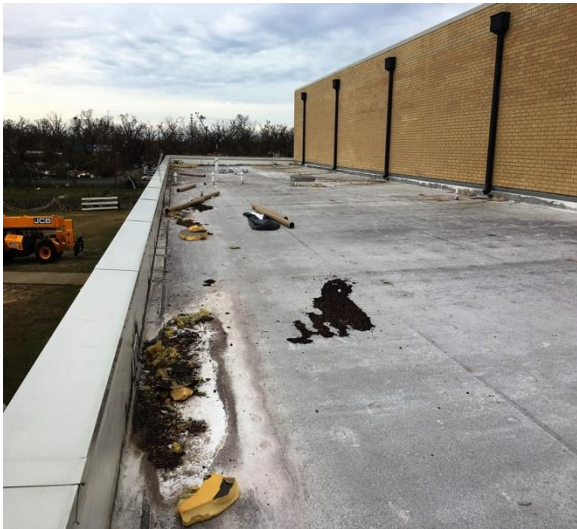
2.1.3 Undamaged lower roof
