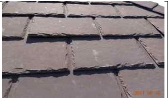
6.07-2. Splash marks on synthetic simulated slate.
