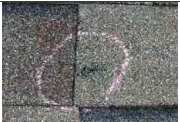
4.04-4. Exposed bitumen in the damaged shingle.
