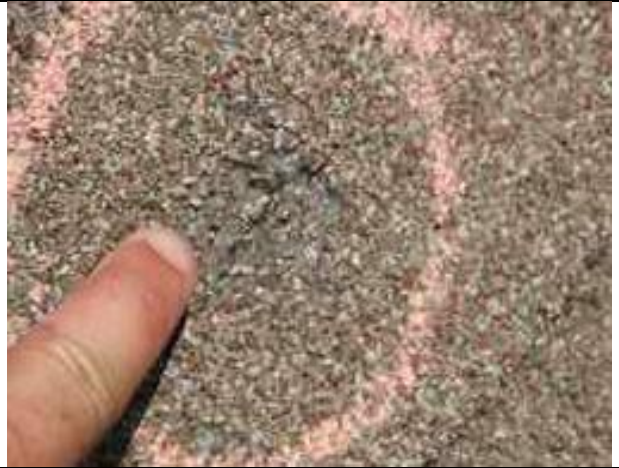
2.06-2. Weathered shingle bruise at ridge.
