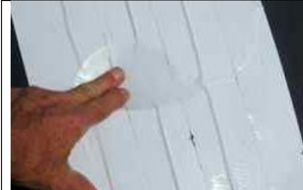
4.03-1. White tape was used as a temporary fix for several skylights that were broken by hail strikes.
