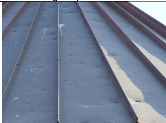
6.15-6. Dents in copper roof panels.
