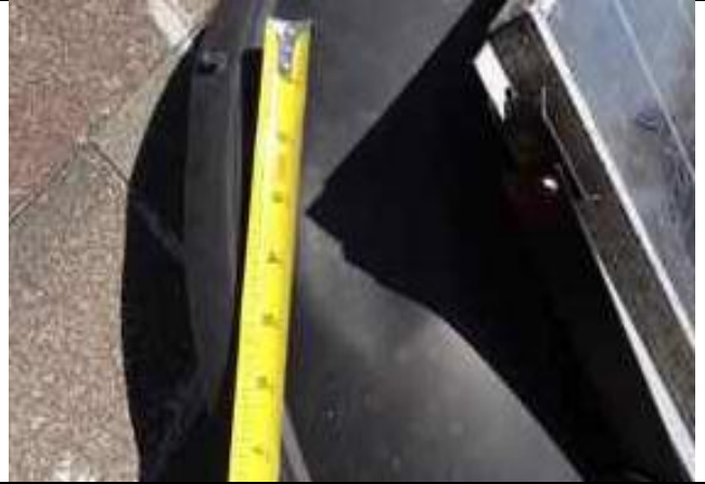
5.18-8. Dent in edge of solar panel vent.
