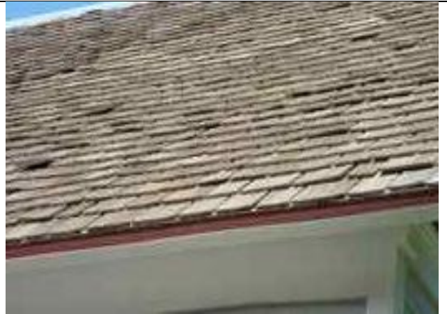
7.02-2. Cedar shingles with some lifting.
