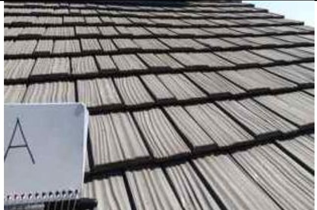
5.15-4. 10' x 10' area on South facing slope with impact locations marked.
