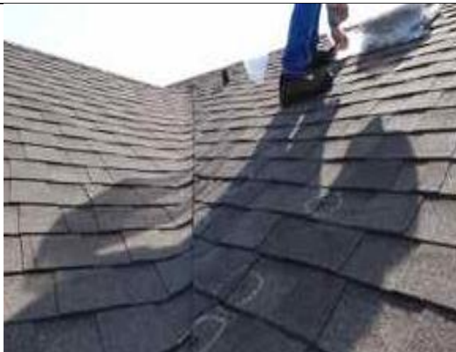
5.12-4. Multiple impact locations along closed-cut valley of IR roof.
