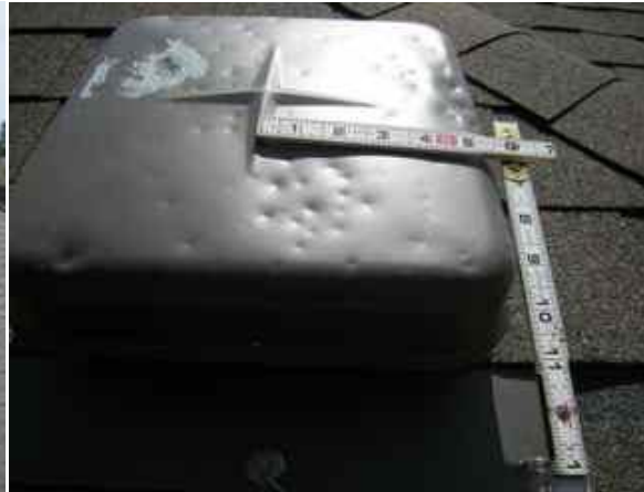
1.03-2. Dents in top of metal vent cover.
