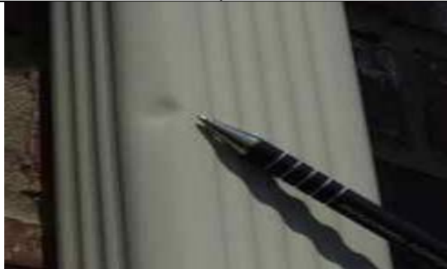
6.13-6. View of a dent in a downspout.
