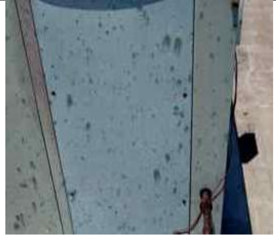
4.08-4. Spatter marks on the side panel of AC unit.
