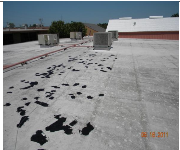
01.20-2. Overview of impact repairs on coated membrane with damage.
