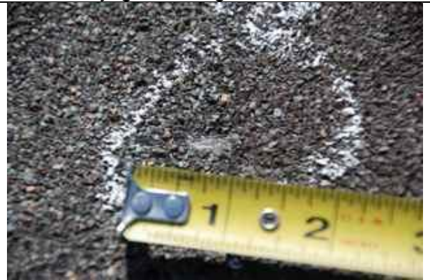
3.07-4 Damage showing reinforcement
