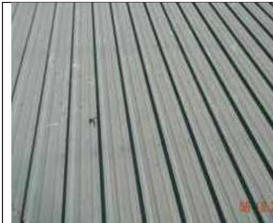
1.16-1. WSW facing slope area with many impact depressions in metal roof ribs.
