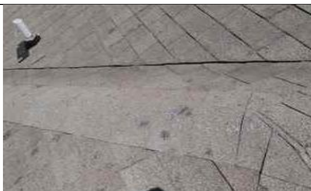
5.06-3. Impact marks on hip shingles.
