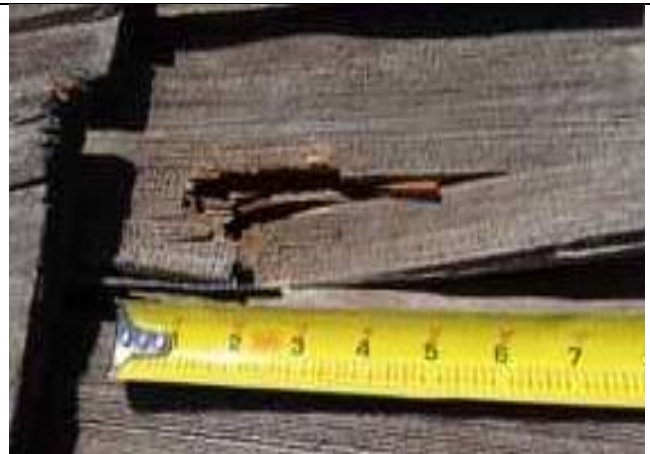
5.17-4. Large impact and broken cedar shake.
