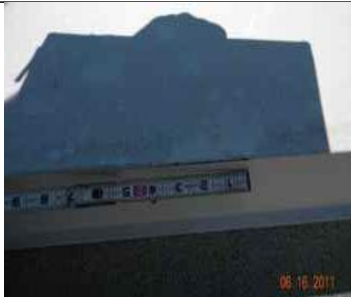
1.19-5. Close-up of impact on coping edge ~ 3-inches.
