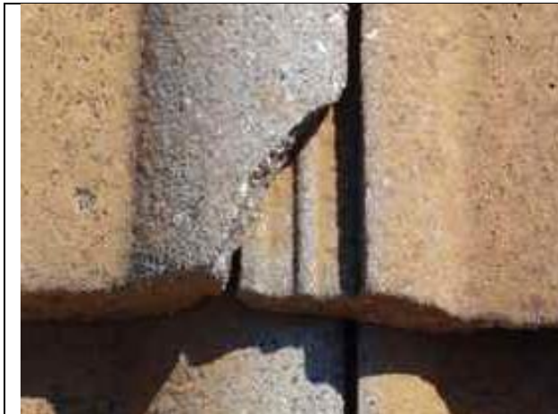
5.16-1. Right corner fracture on concrete barrel tile.
