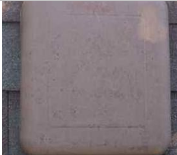
6.11-3. Splash marks on steel attic vent.
