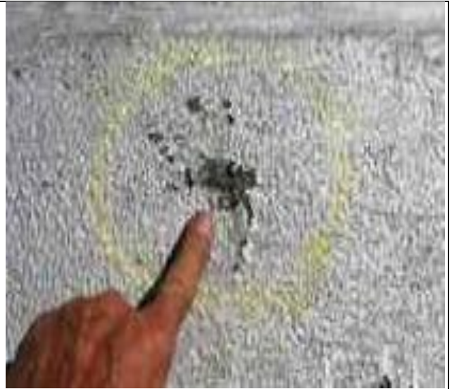
4.09-2. Chipped aluminized coating on the base/wall flashing.
