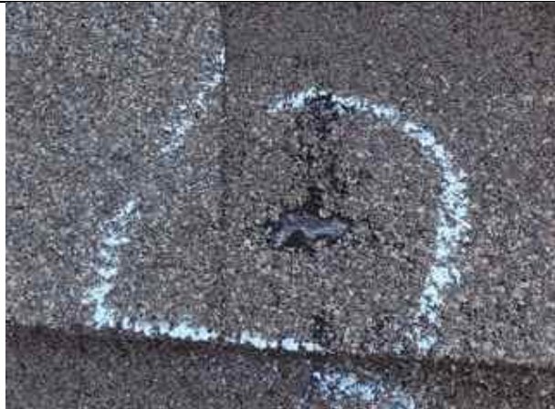
5.11-3. Hail damage showing felts
