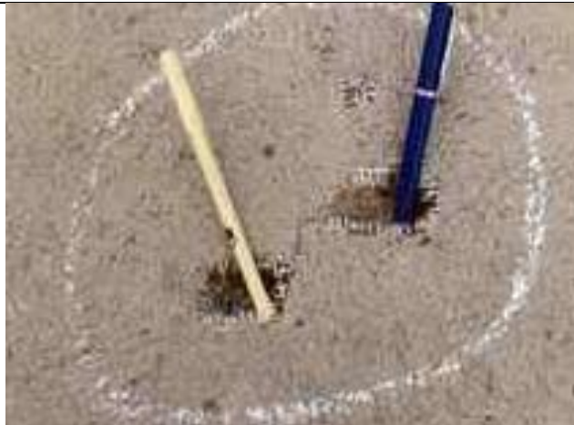
4.02-3. This is a close-up of two holes in the EIFS consistent with hail strikes.
