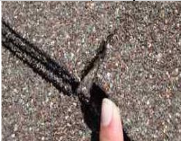
5.18-3. Tear on shingle edge.
