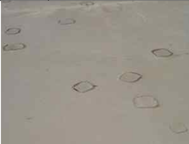
7.03-3. Repaired punctures on flat roof.
