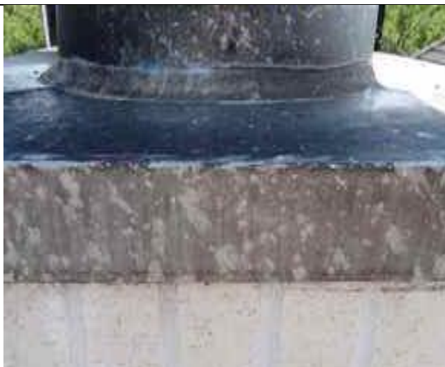
5.12-2. Splatter marks on chimney vents.
