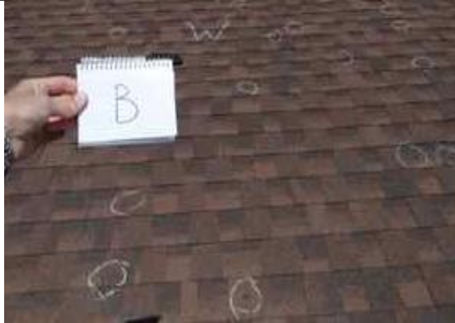
5.07-7. Impact locations marked on West facing slope of roof.
