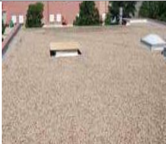
3.10-3. Damaged skylight and no visible damage to BUR.
