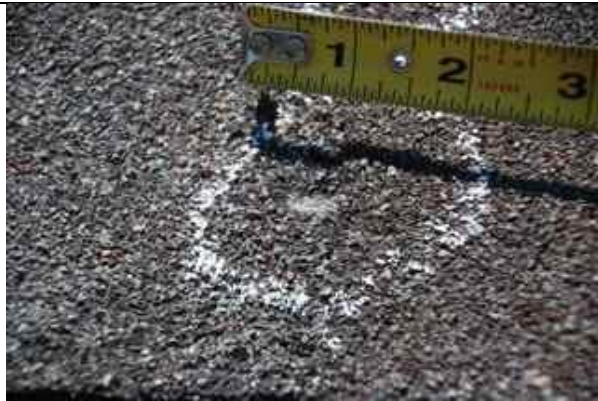
3.07-3 Damaged shingle
