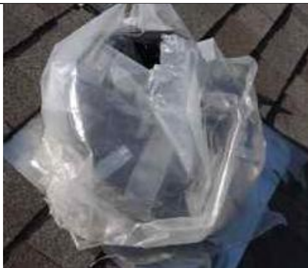
5.12-1. Severe damage to plastic static roof vent.
