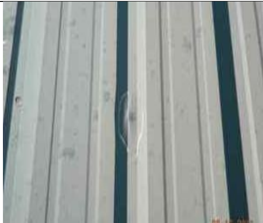
1.16-3. Overview close-up of impact depressions in metal roof rib.
