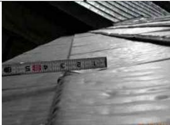
1.23-3. Metal damage from hail.
