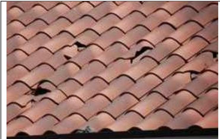
3.12B-1. Typical tile roof damage due to hail impacts at this site.
