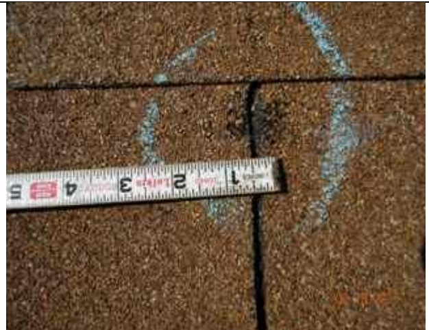
1.14-2. Overview of 1-inch impact mark on damaged 3-tab shingle.
