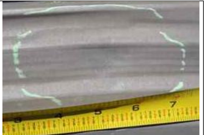
5.15-2. Large dent in metal shingle.
