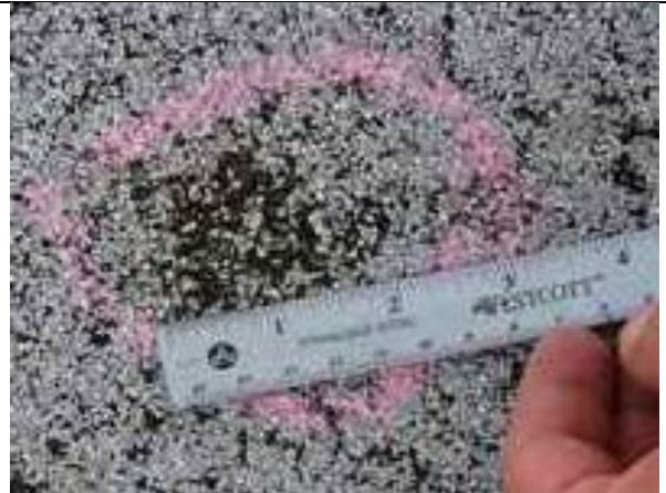
4.06-6. Displaced granules on the surface of the mod. bit roof.
