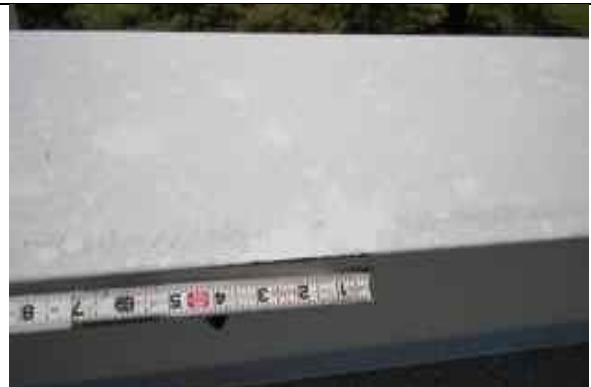
1.19-4. Close-up of impact on coping edge ~ 3-inches.
