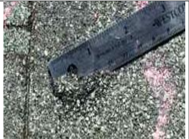
4.05-2. Fractured laminated shingle.
