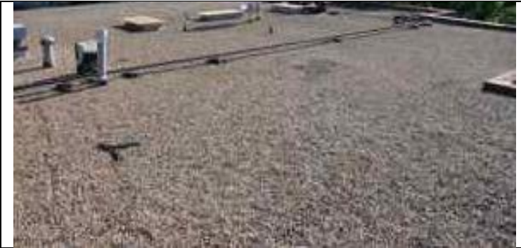
3.08B-1. Hail impact divots in BUR roof.
