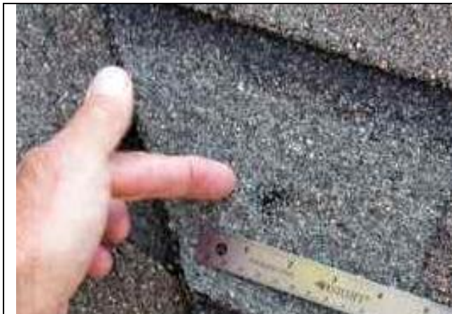
4.04-1. Possible hail damage on class 4 shingles.
