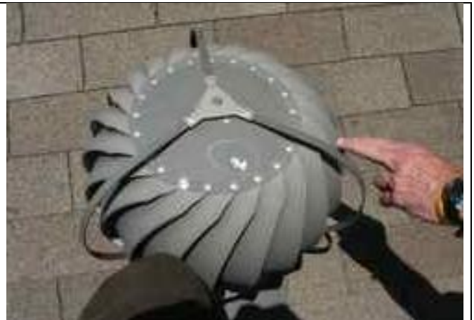
2.07-2. Dent in aluminum turbine vent.
