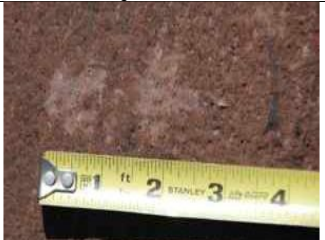
3.11-4. Typical hail splatter mark on tile.
