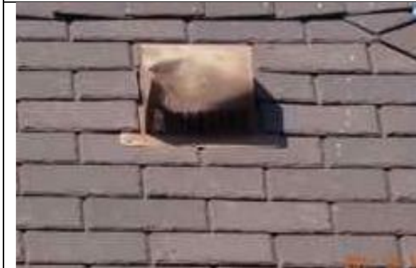
6.07-3. Dent on attic vent.
