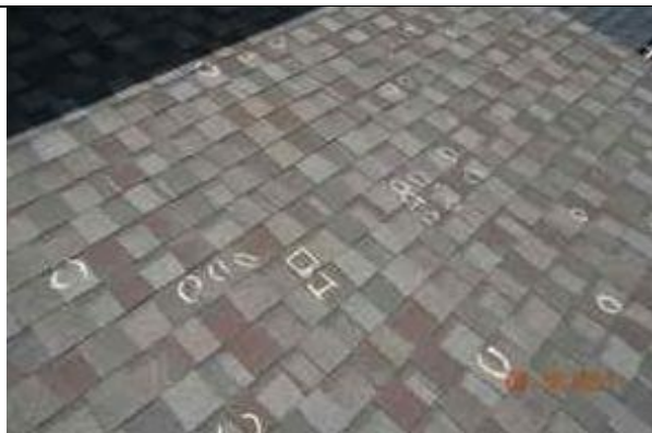
1.11-1. West facing slope area with many impacted shingles.
