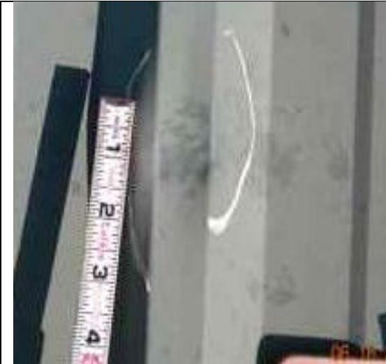
1.16-5. Overview close-up of impact depressions in metal roof rib.
