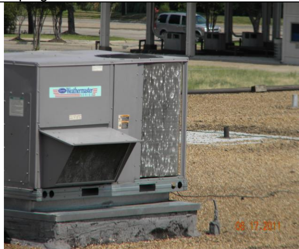
01-26.4. Hail-caused dents to RTU fins.
