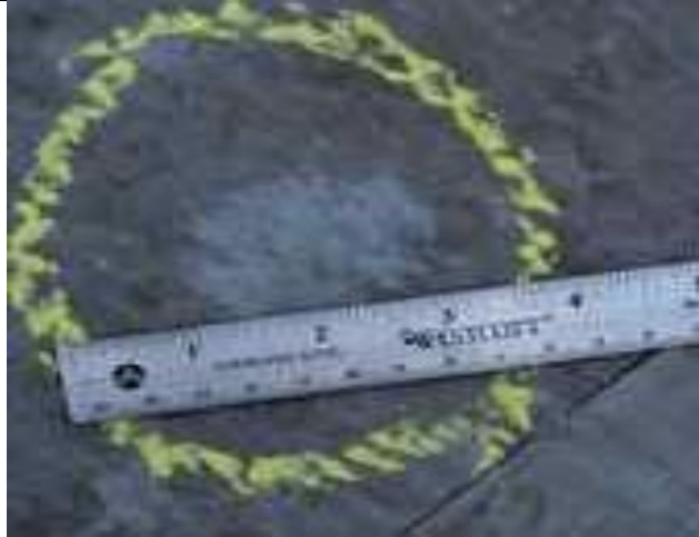
4.08-3. Spatter mark on the wall flashing.
