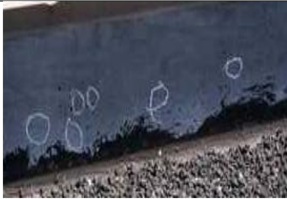
4.03-5. Encircled on the wall/base flashings of this parapet are numerous hail strike locations.
