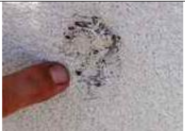
4.06-2. Close-up picture of the punctured EIFS wall surface.
