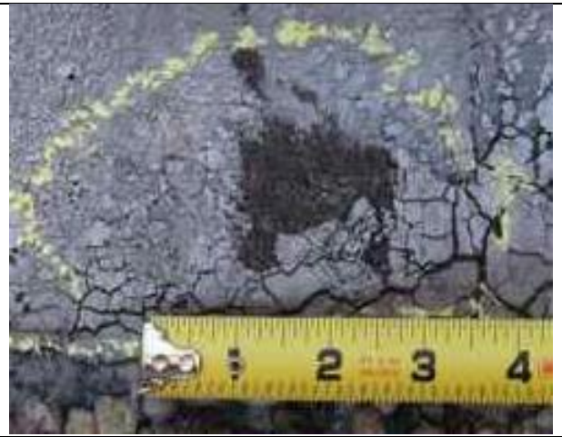
4.10-6. Chipped aluminized coating on the base flashing.
