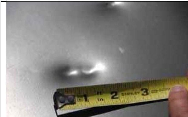
3.09-1. Hail impact dents in metal flashing on top of parapet wall.
