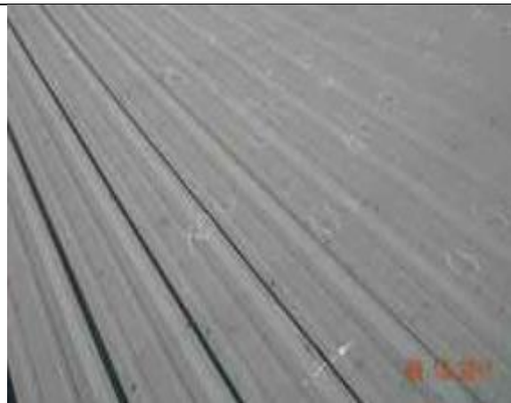
1.16-2. WSW facing slope area with many impact depressions in metal roof ribs. Overview of impact marks (circled on metal panels).
