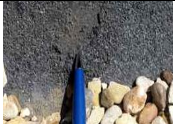
4.02-6. Close examination of this base flashing showed bare spots where mineral granules were knocked loose.
