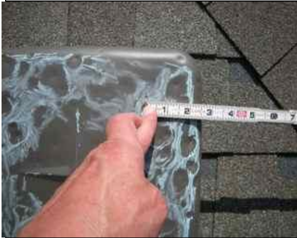
1.03-3. Dents in top of metal vent cover after chalk-rub.
