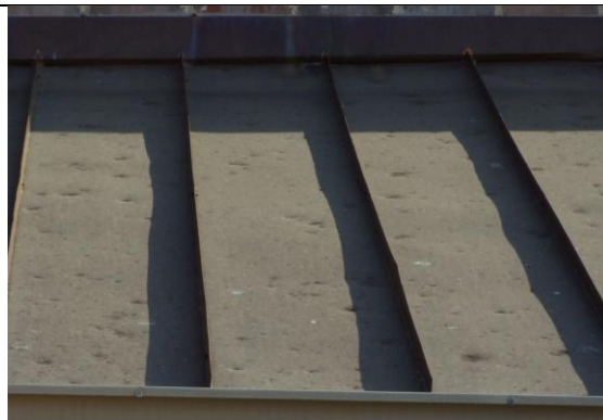
6.15-2. Dents in copper roof panels.
