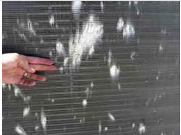
4.06-4. Indentation on the heat exchanger fins on roof mounted AC unit.
