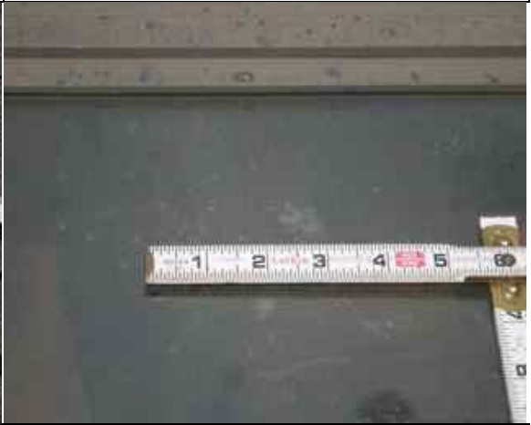
1.03-4. Hail spatter mark on horizontal glass pane of skylight.
