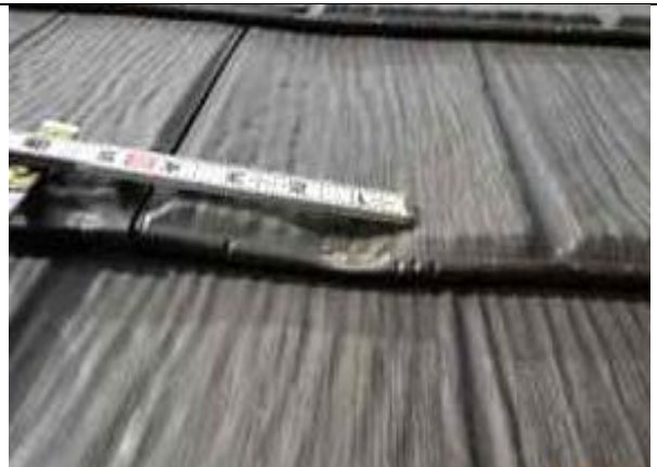
1.23-4. Shingle damage from hail.
