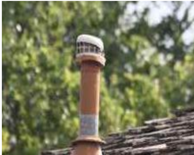
7.06-3. Damaged hot vent cap.
