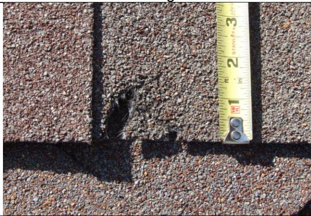
6.11-7. Penetrating damage with erosion
