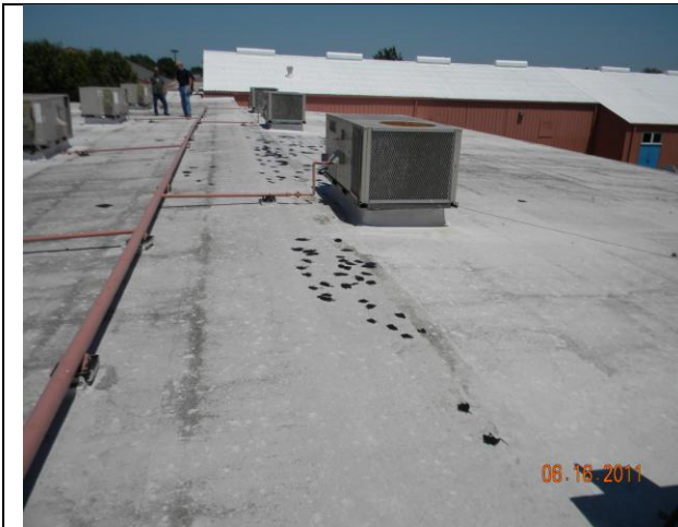
01.20-1. Overview of impact repairs on coated membrane with damage.
