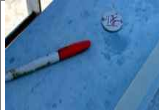
4.08-1. Spatter marks on the metal coping.
