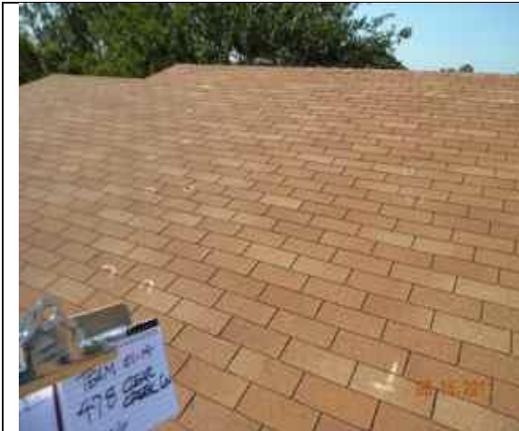
1.14-1. South facing slope area with many impacted shingles.
