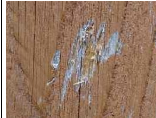
5.17-3. Splatter mark on stained wooden fence.
