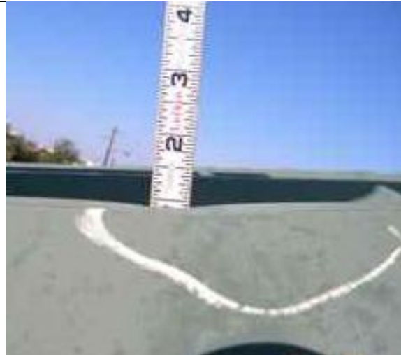
1.16-6. Cross view close-up of impact depressions in metal roof rib.
