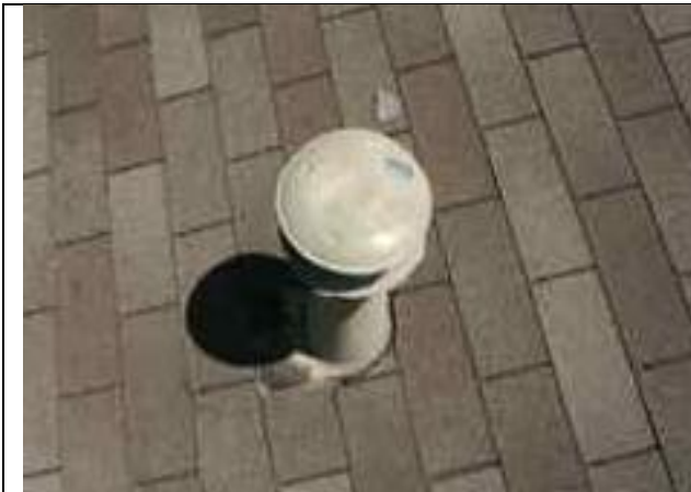
2.07-1. Dented flue cap.
