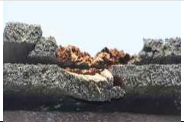
7.06-2. Damage to starter course wood shake.
