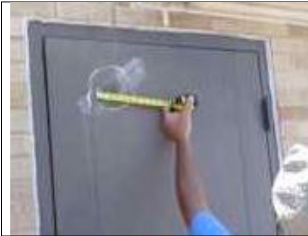
4.10-5. Indentation on the metal door apparently caused by a large hailstone.
