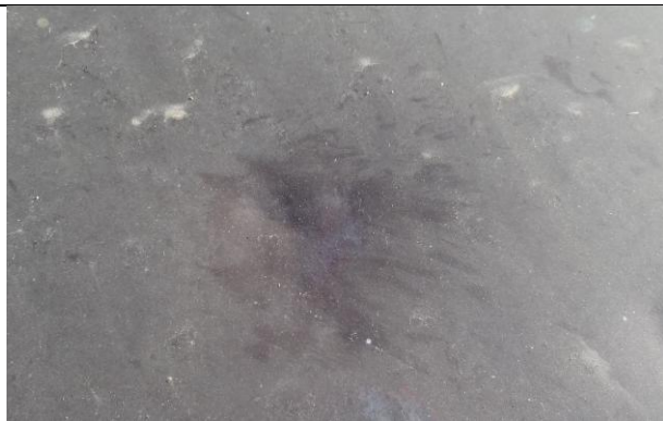
6.15-1. Splash mark and dent on copper roof panel.
