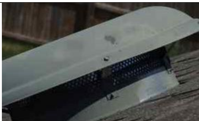
6.13-2. View splash mark on an attic vent.
