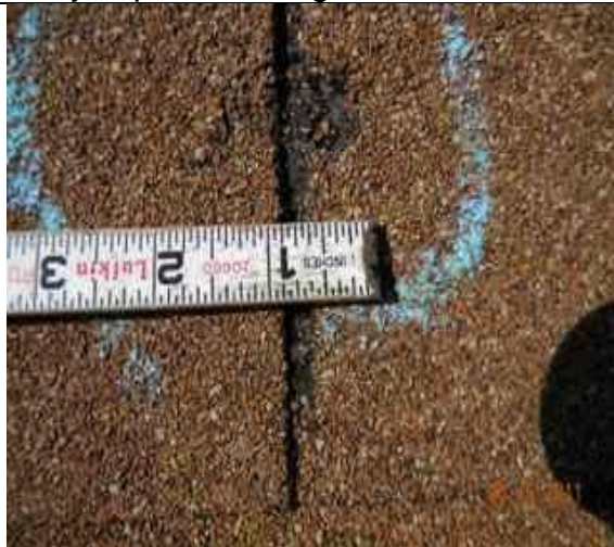
1.14-3. Overview of 1-inch to 1-1/4-inch impact mark on damaged 3-tab shingle.
