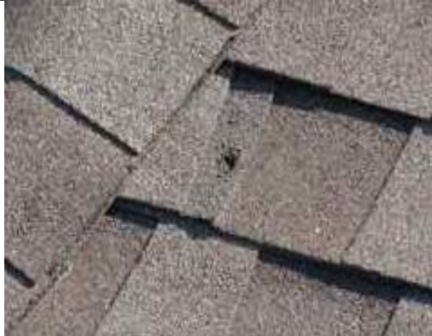
5.12-5. Puncture on IR shingle.
