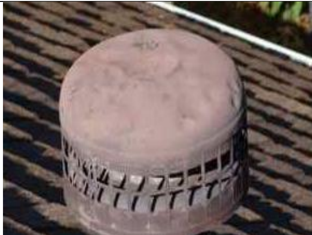
5.14-3. Dents and splatter marks in metal vent.
