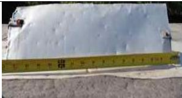
5.13-3. Numerous impacts in metal chimney cover.
