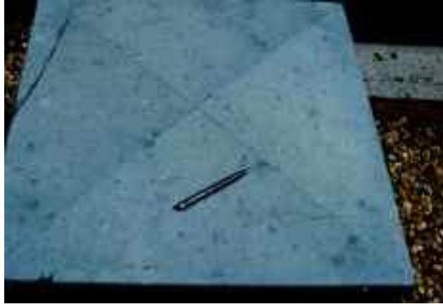
4.02-1. The dark spots on top of this sheet metal cap are spatter marks from hail strikes. The larger ones appear to be from hailstones of 1"–1.25" diameter.
