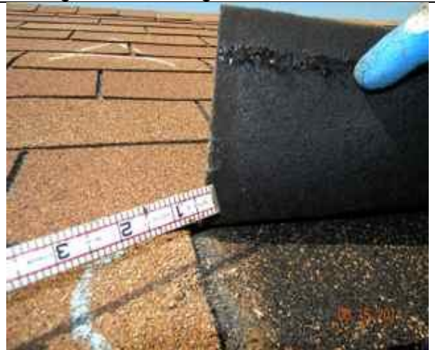
1.14-4. Damaged 3 tab shingle in Photo 5.
