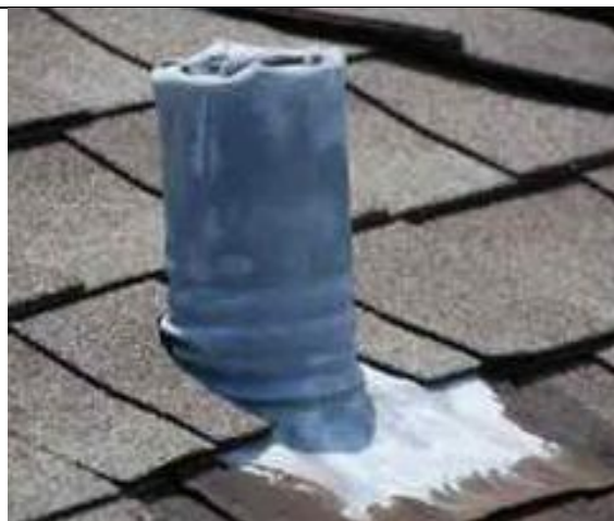
3.03-4. Same vent stack at 3.03-3 indicating damage on opposite side.
