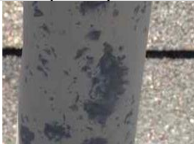
5.18-4. Spatter marks on metal vent stack.
