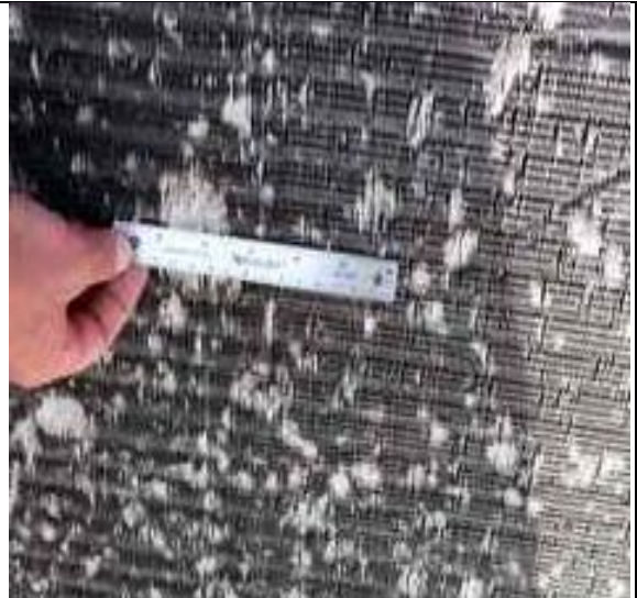
4.08-6. Indentations on the heat exchanger fins on roof mounted AC unit.
