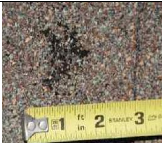
3.03-2. Typical hail damage for this site.
