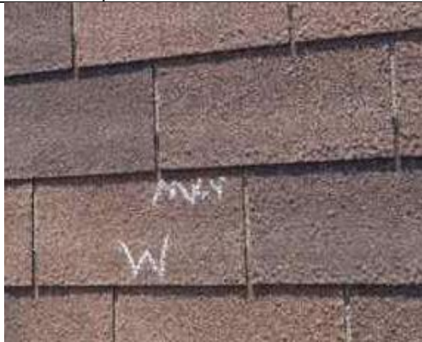
5.01-3. West facing slope, IR blisters.
