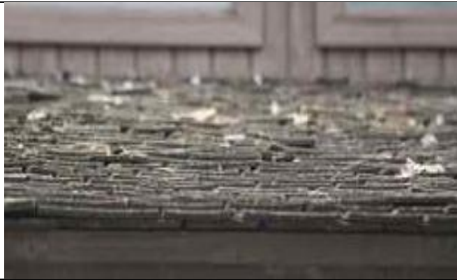
7.06-1. Broken shakes scattered as debris.
