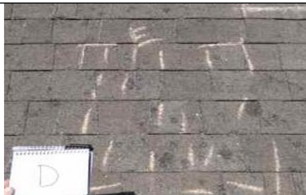
5.06-2. Measured areas with impact locations marked on East facing slope.
