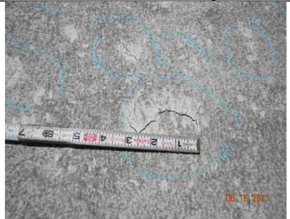
01.20-4. Close view of impact damage ~ 3 to 3.5-inch.
