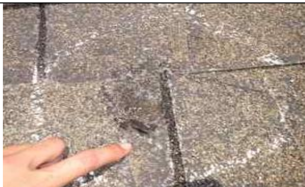
5.06-1. Impact fracture on shingle tab.
