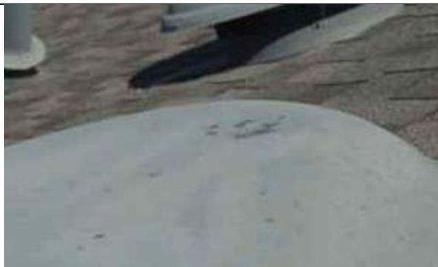
6.13-3. View splash mark on an attic vent.
