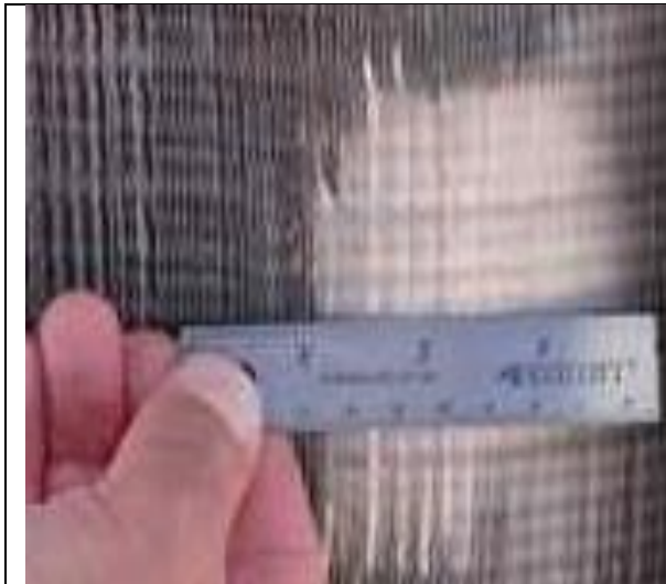
4.09-5. Multiple indentations on the heat exchanger fins on roof mounted AC unit.
