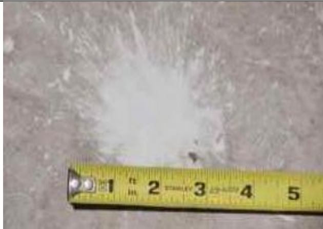
3.12-3. Typical large hail strike to single ply roof covering. Would need core sampling to determine underlying damage at this site.
