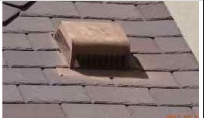
6.07-4. Splash marks on attic vent.
