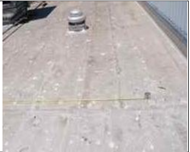
3.12-2. Large number of big hail strikes to single ply roof covering at this location.
