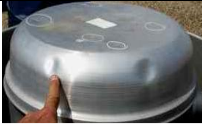
4.02-5. Several indentations (encircled in white) were noted on this exhaust cover.
