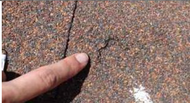
5.07-9. Close-up of impact fracture on shingle.
