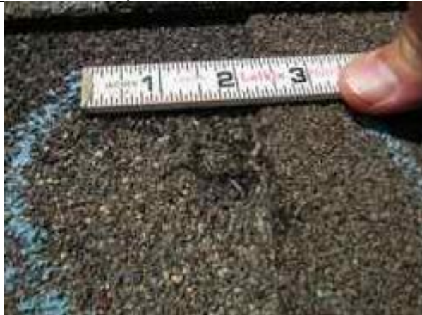
1.06-3. Hail damage on shingle.
