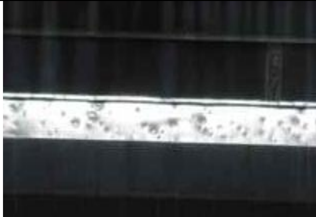
4.11-1. Multiple indentations on the copper gutter.
