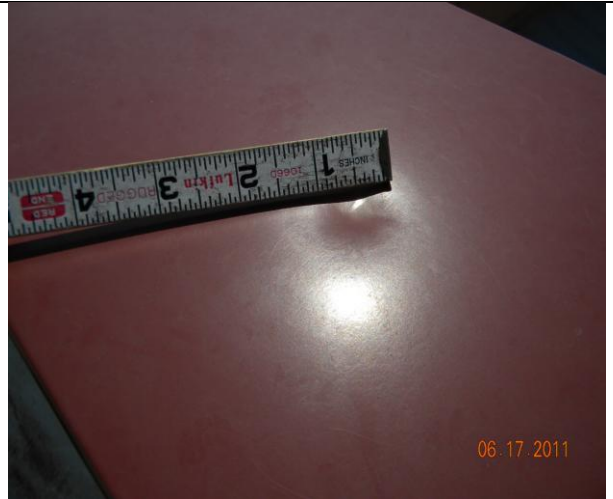
01.26-2. Close view of impact damage in coping ~ 1-inch.
