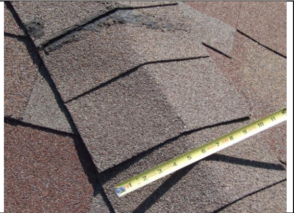
6.11-6. Crack in unsupported area
