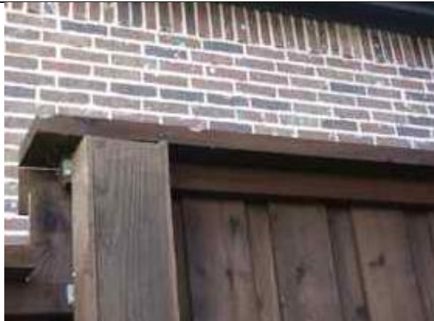
6.14-3. View of chipped wood on the top rail of a wood fence.
