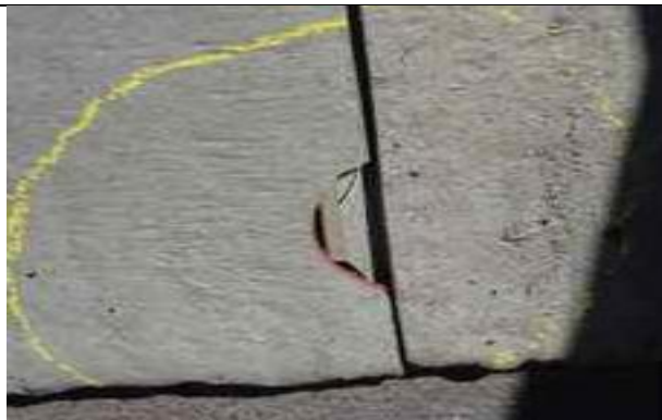
4.11-3. Chipped edge of tile on steep slope roof.
