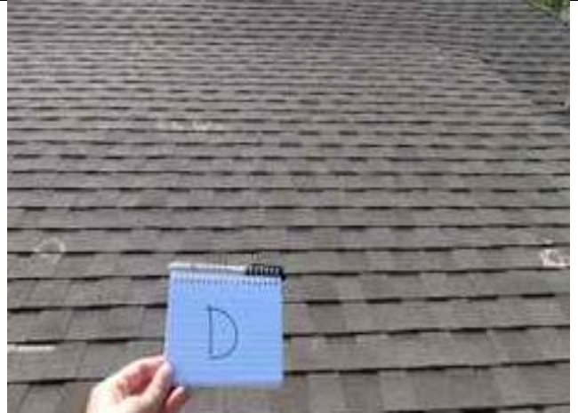
5.12-6. 10' x 10' area on West facing slope with impact locations marked (IR roof).
