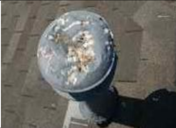
2.09-3. Dented flue cap.
