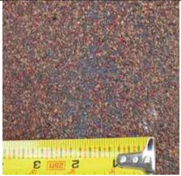
5.03-2. Damage mark from hail.
