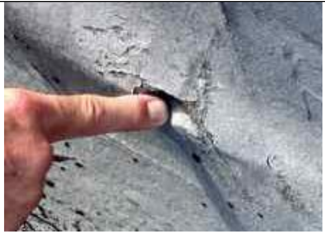
4.03-4. This is a close-up view of racked felts on a parapet with evidence of hail strikes.
