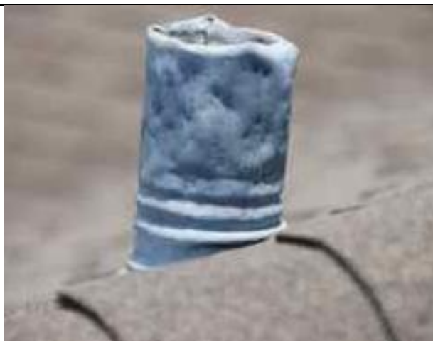
3.03-3. Dents on vent stack indicating hail impact from southwest.
