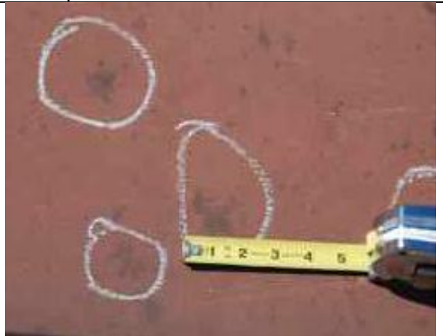
3.10-4. Typical hail impact damage to parapet cap flashing.
