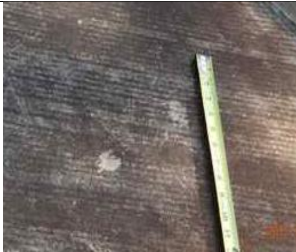
6.01-3. Splash marks on steel chimney cap.
