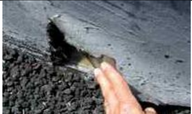
4.03-2. The old, weathered felts on this wall were especially vulnerable to damage from hail strikes
