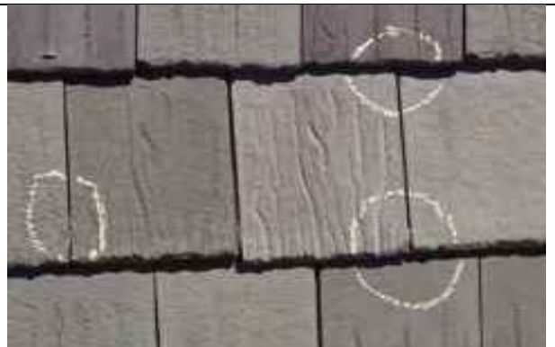
4.11-4. Multiple chipped tiles on steep slope roof.
