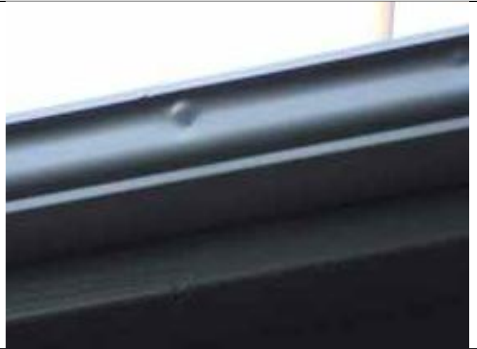
6.14-2. View of dents in a gutter.
