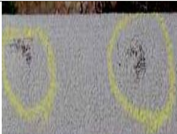
4.06-9. Puncture marks on the EIFS surface.
