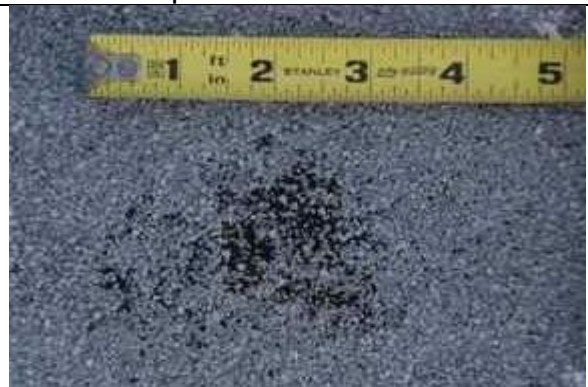
3.09-4. Typical hail impact damage to roof.
