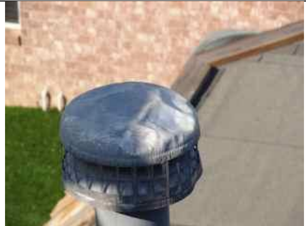
5.11-4. Hail damage on vent stack
