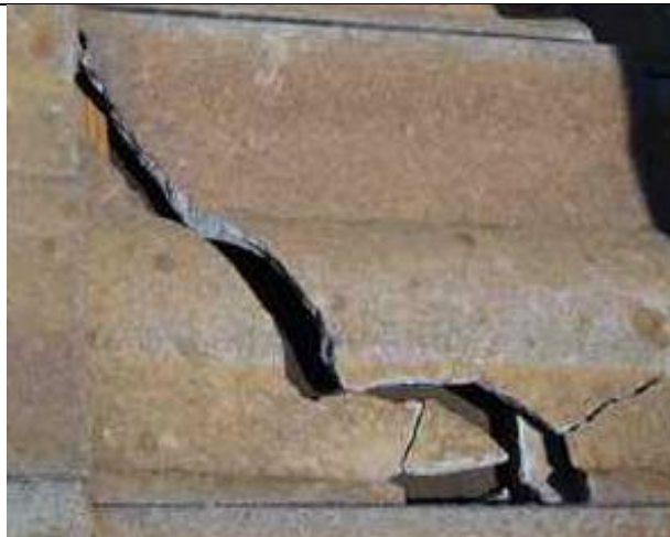
5.16-3. Fracture from large hail impact.
