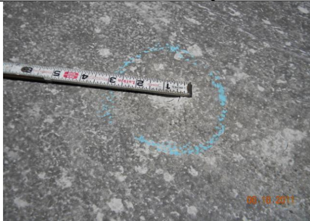
01.20-3. Close view of impact damage ~ 1.5-inch.
