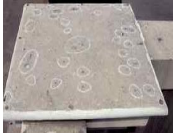
4.02-2. At the SW and NW corners of this roof are square enclosures lined with walls, and the walls are topped with exterior insulation and finish system (EIFS).
