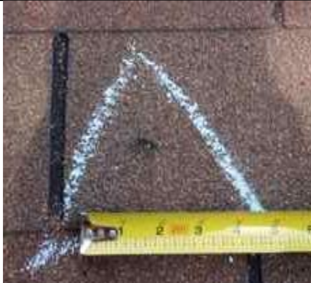
5.03-1. Damage mark from hail.
