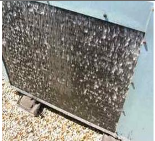
4.09-4. Multiple indentations on the heat exchanger fins on roof mounted AC unit.
