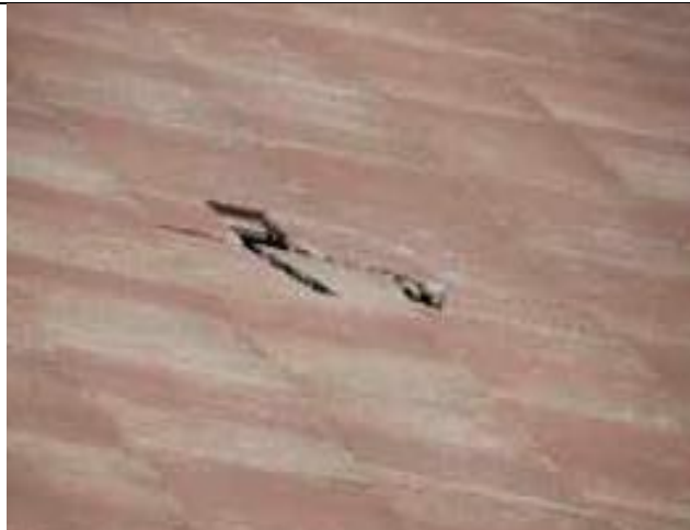
3.11-3. Tile fractured. Note white "splatter" marks indicating hail impact.
