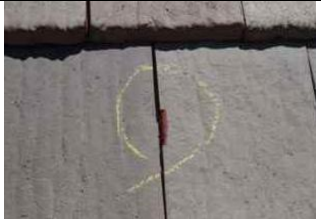
4.11-2. Chipped edge of tile on steep slope roof.
