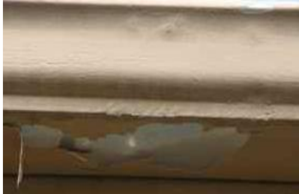
2.19-9. Dented gutter.
