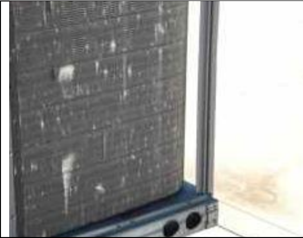
7.03-1. Damaged rooftop unit impacted by hail sideways.
