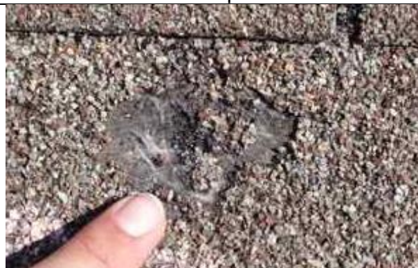
5.09-6. Damaged shingle.
