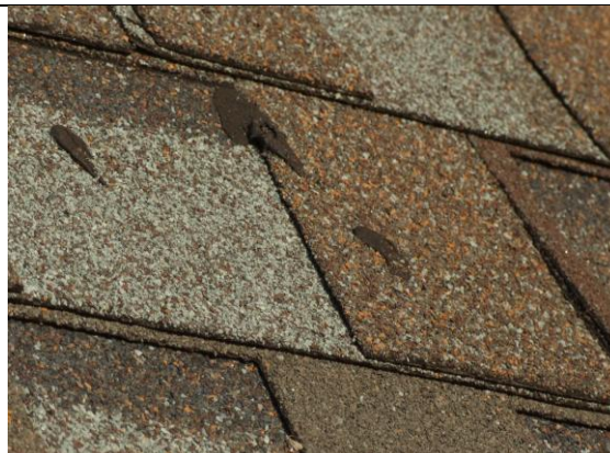
6.15-4. Shingle repairs unrelated to hail.
