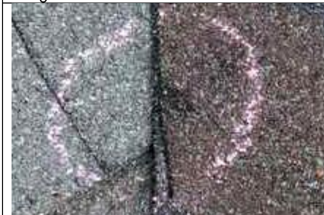
4.04-3. Exposed bitumen in the damaged shingle.
