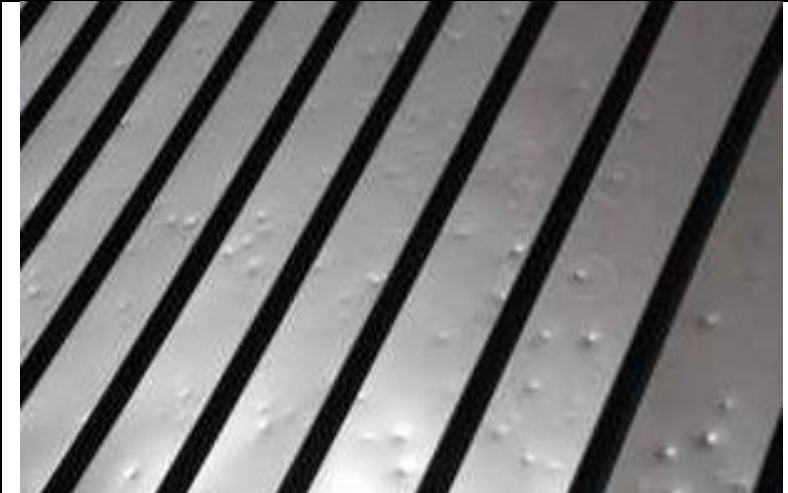
3.09B-1. Dents in standing seam metal roof from hail impact.
