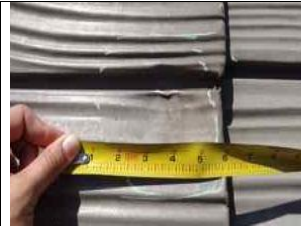
5.15-1. Large dent in metal shingle.
