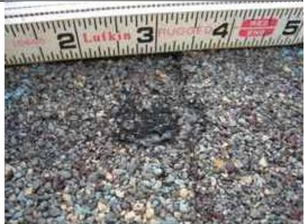
1.06-4. Hail damage on shingle.
