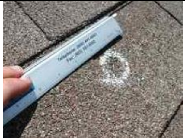
7.05-2. Hail-caused bruise on asphalt shingle.
