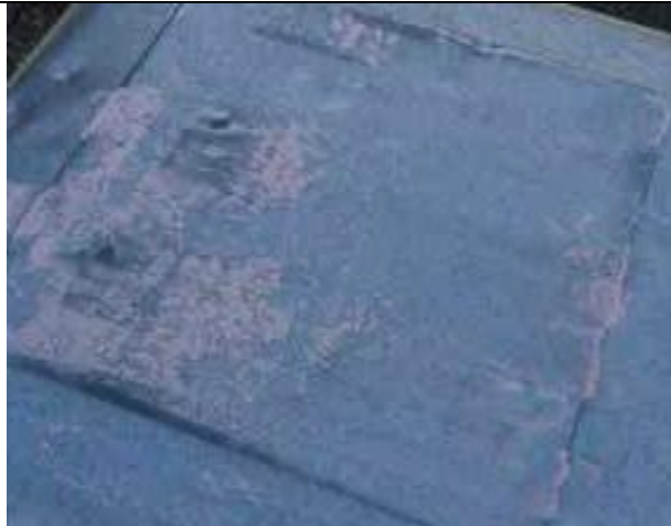
5.12-7. Dents in metal roof vent highlighted by chalk.
