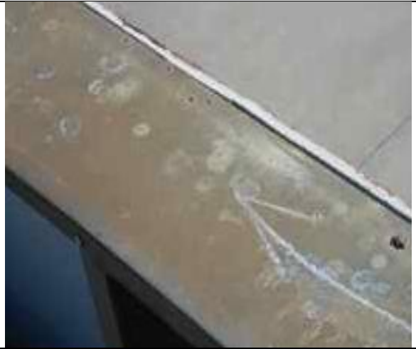
7.03-2. Pockmarks on parapet.
