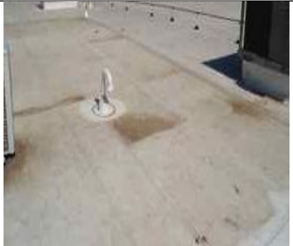
7.03-4. TPO and PVC on same roof.
