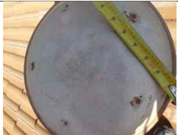
5.16-2. Large dents in metal vent.
