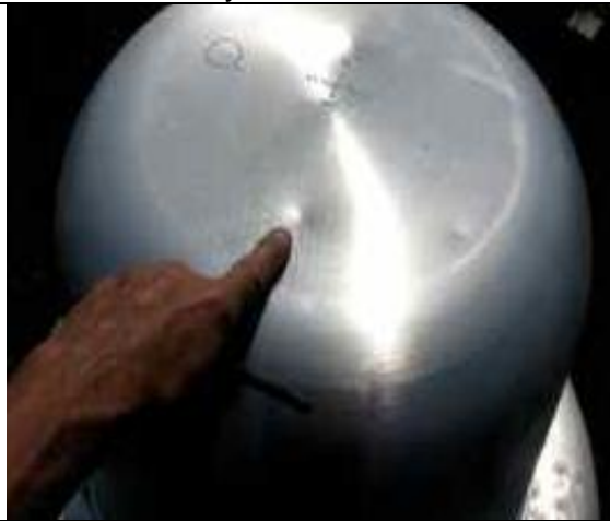
4.03-3. Sheet metal exhaust units provide conspicuous evidence of hail strikes.
