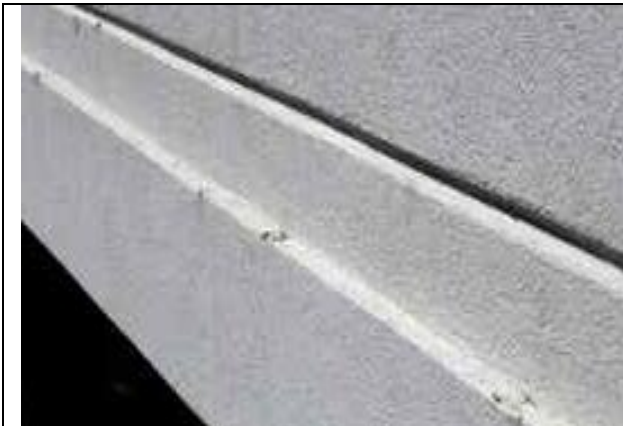
4.06-1. Puncture marks on the EIFS wall.
