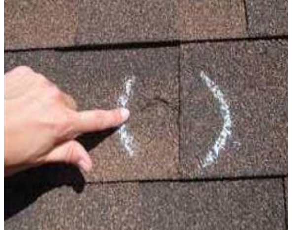
5.07-8. Impact fracture on face of shingle.
