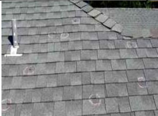
4.05-3. Several damaged asphalt shingles on the roof.
