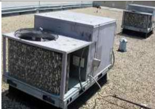
4.02-7. Cooling fins on both of these HVAC units show widespread damage from hail strikes.
